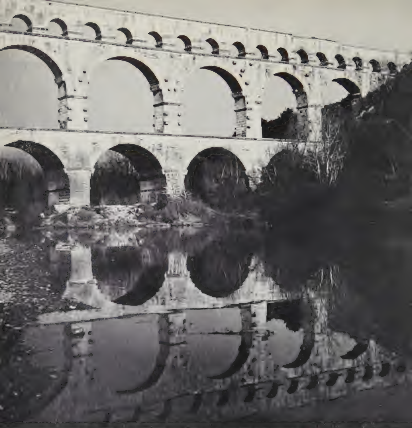
Pont du Gard, a Roman aqueduct which for centuries brought water to Nimes, France
